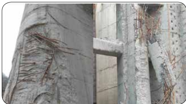
Damage on Barrage Pier and Intake structure
